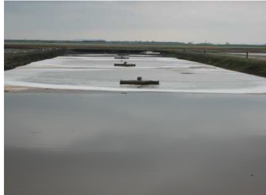
Day 120 Sludge Level 3'
