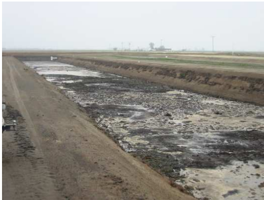
Day 0 Sludge Level 15'
