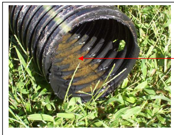
Flooded Drainfield
