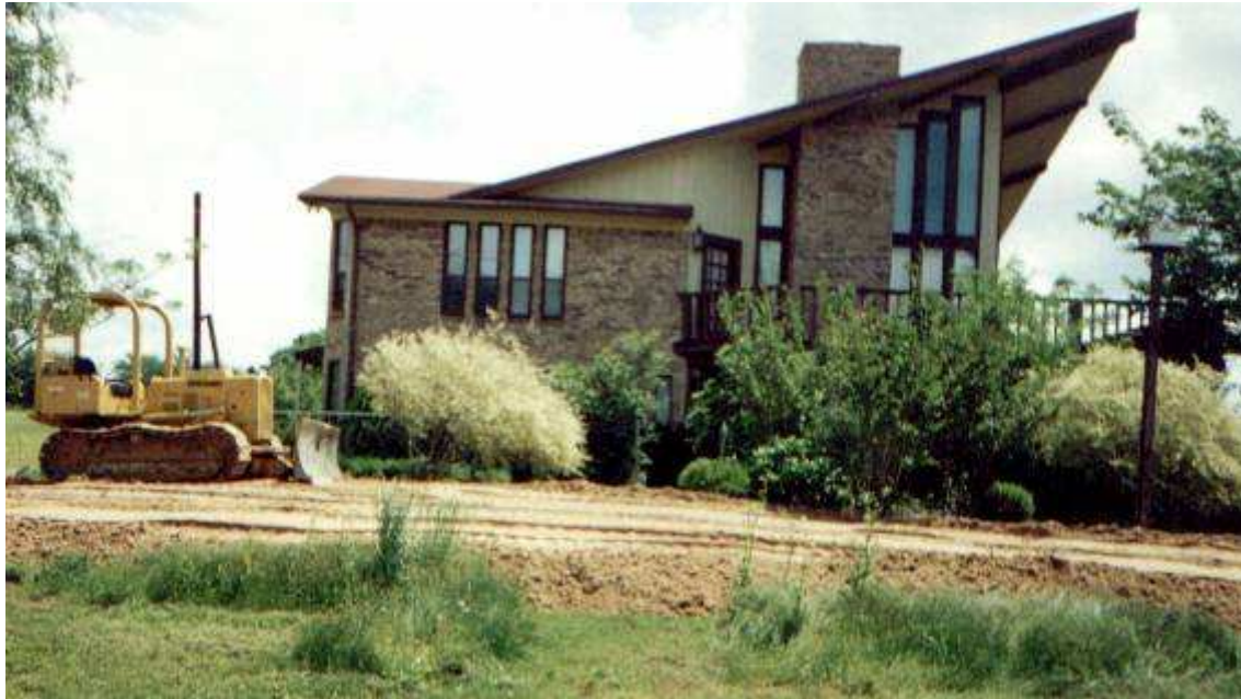
Figure 6. Remediation of a 100% failed system at the Hogue site.
