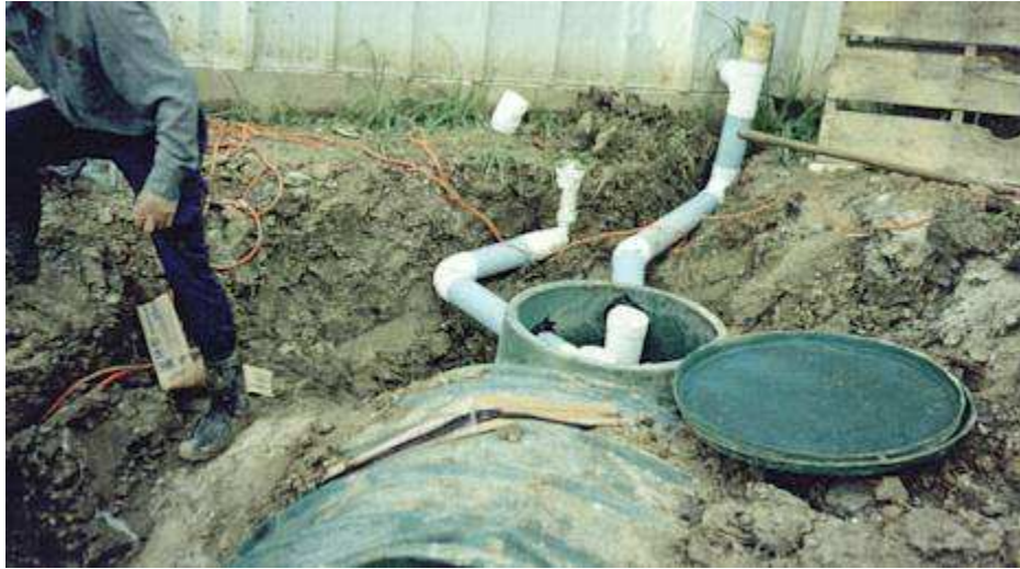
Figure 1. Initial excavation and emplacement of a 1250-gallon digesting tank at LoneStar Charlie's.
